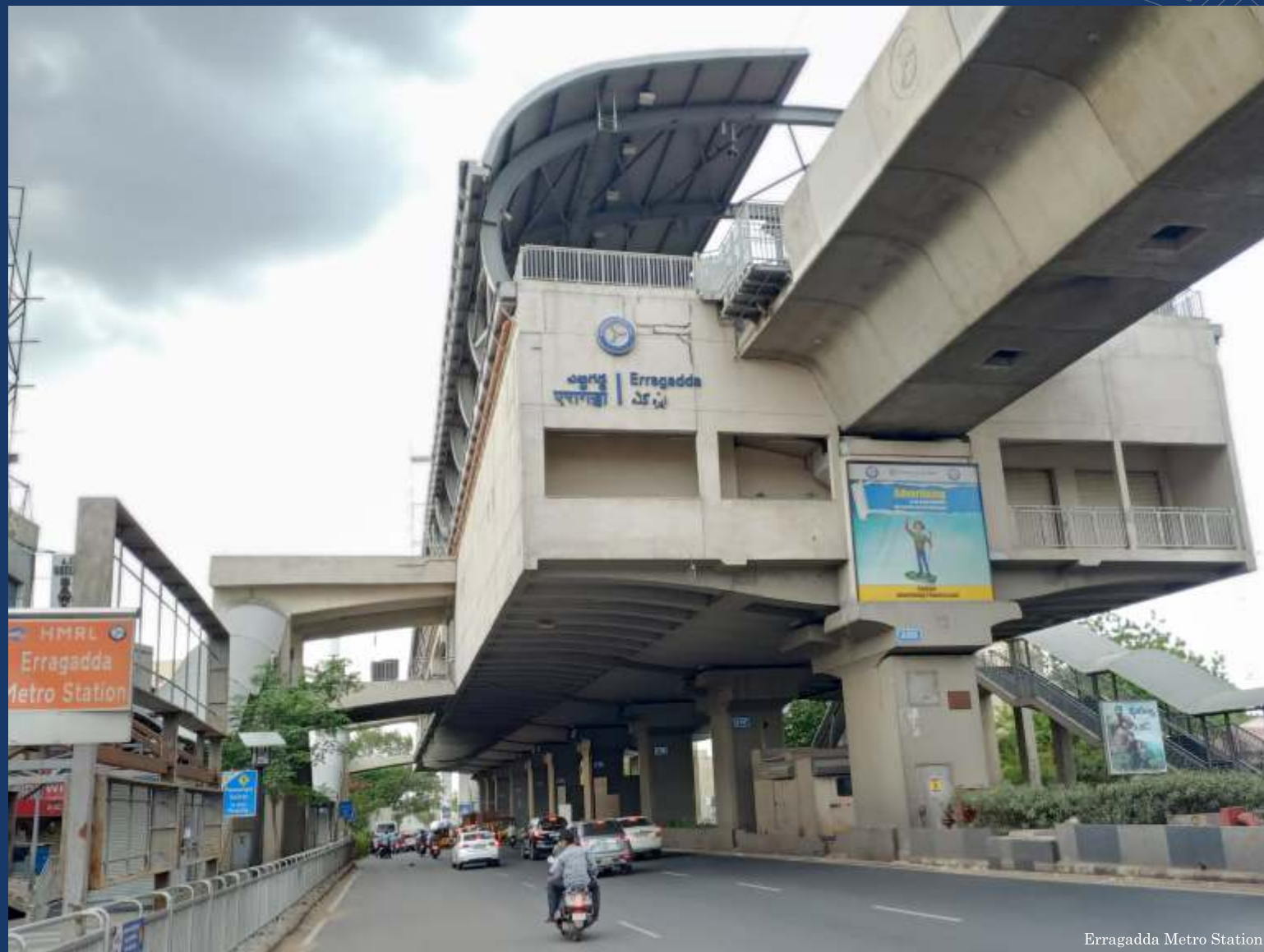
Erragadda Metro Station
